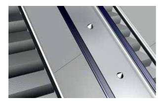
Figure 6.6 Anti-slide cones
